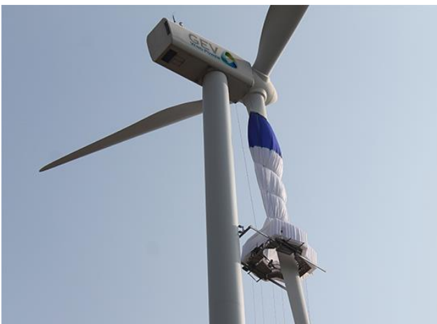
Figure 20: GEV blade repair system
